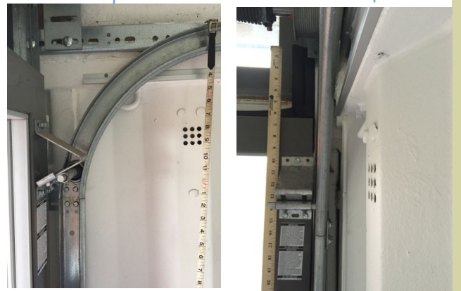
Views of Top of Door in Need of Light-Blocking Solution
